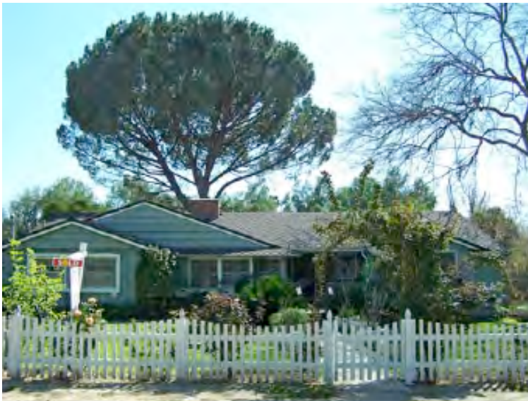
Figure 31 – Site Photo 4 by Author.
