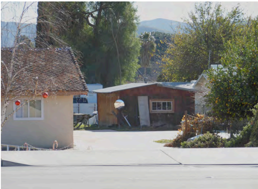
Figure 37 – Site Photo 10 by Author.
