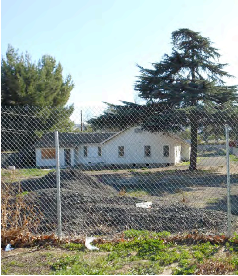
Figure 36 – Site Photo 9 by Author.
